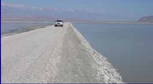
Containment berms and ponds
